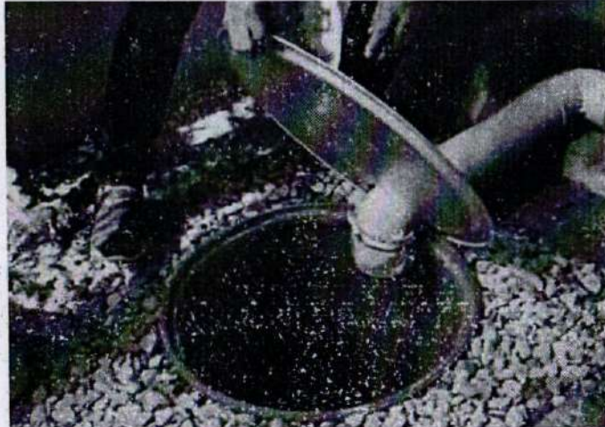
08) Covering Pipe with Cloth for filtration
