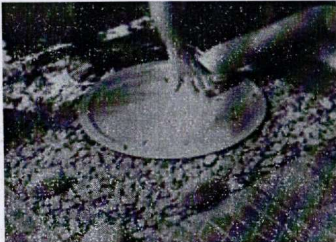
07) Gravel Filling at Periphery and inside entire pit and covering it from top with lid
